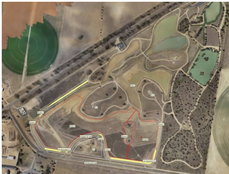
Figure 7: Aerial view of the Narromine Wetlands Project
