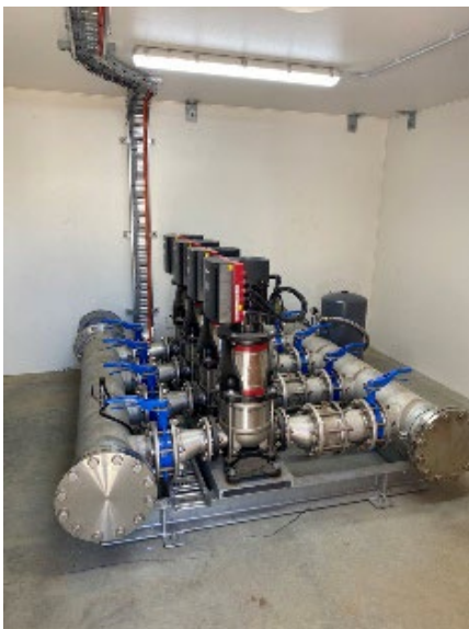
Figure 1: The new booster pump station on Duffy Street, Left: pump skid, right: electrical switchboard
