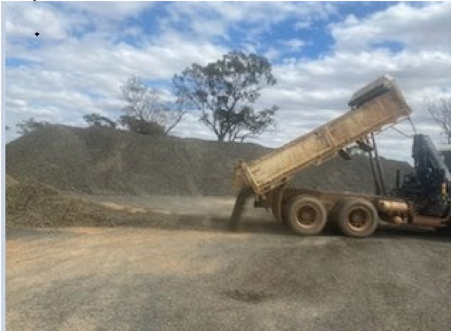
Figure 12: Carting material to a job site
