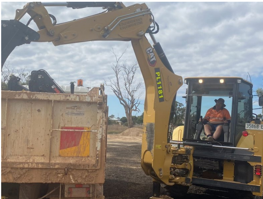
Figure 13: Council's roads team utilising the excavator.
