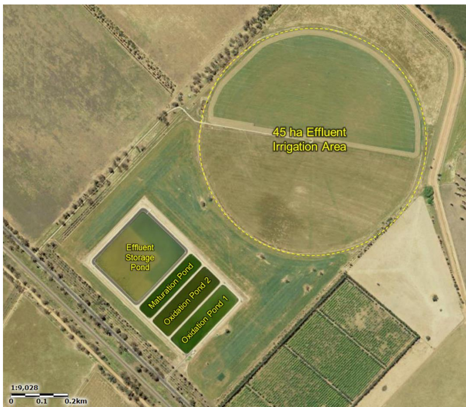
Figure 12-3: Narromine STP aerial photo
