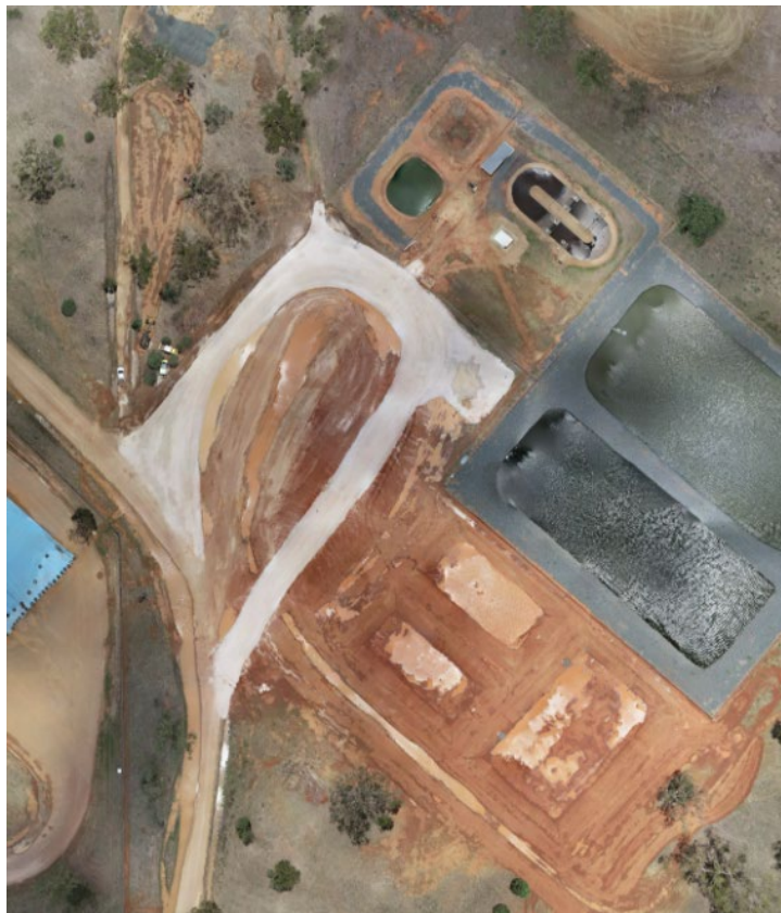
Figure 14: Aerial view of Trangie Truck Wash
