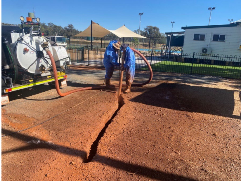
Figure 4: Staff using the new excavation trailer at Tomingley
